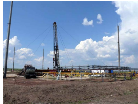
VM#1 well workover in operation
