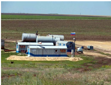
VM field site office
