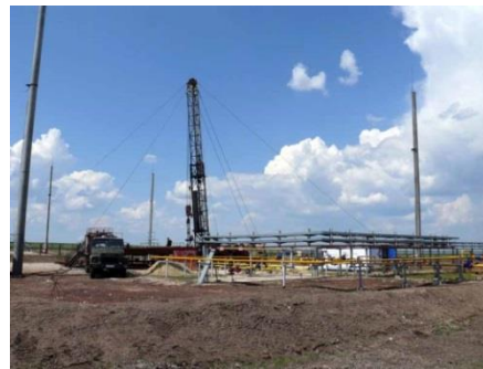
VM#1 well workover in operation
