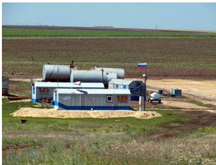
VM field site office
